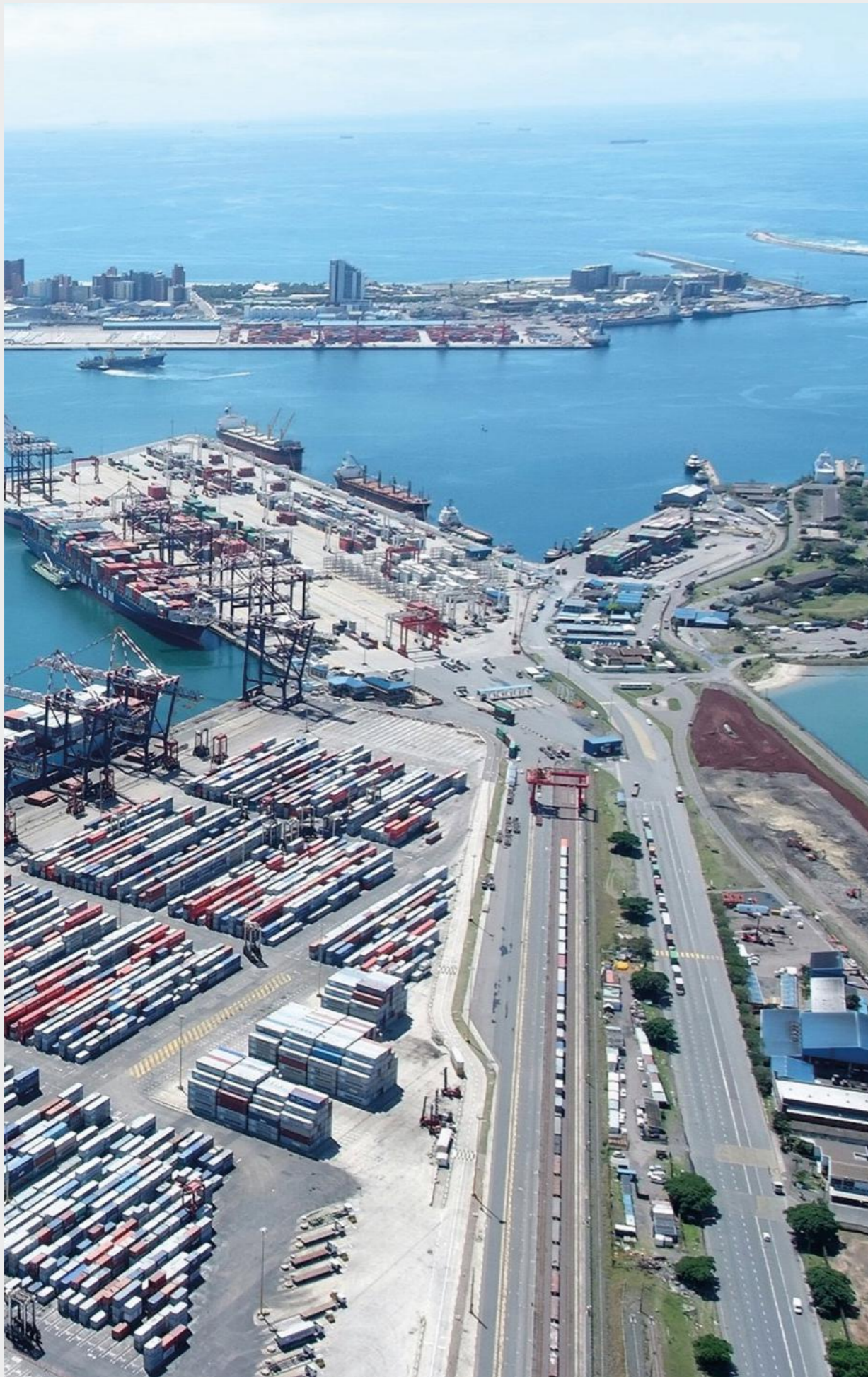
Port of Durban Z-shape Durban Container Terminal Piers 1 and 2
