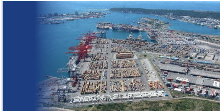
A view of the Durban Container Terminal 1
