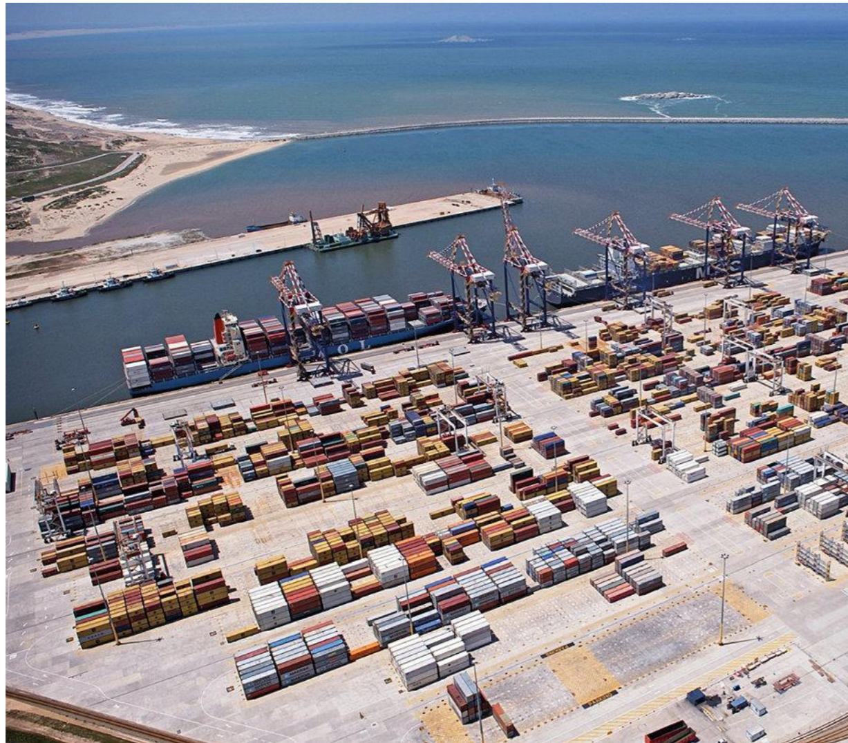
Ngqura container terminals
