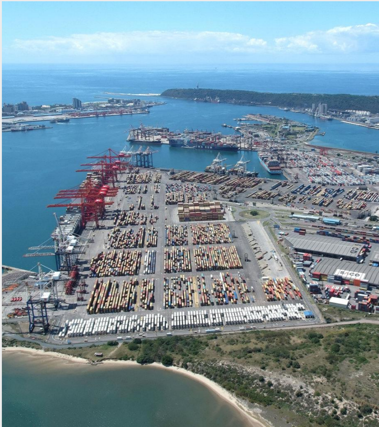
A view of the Durban Container Terminal 1
