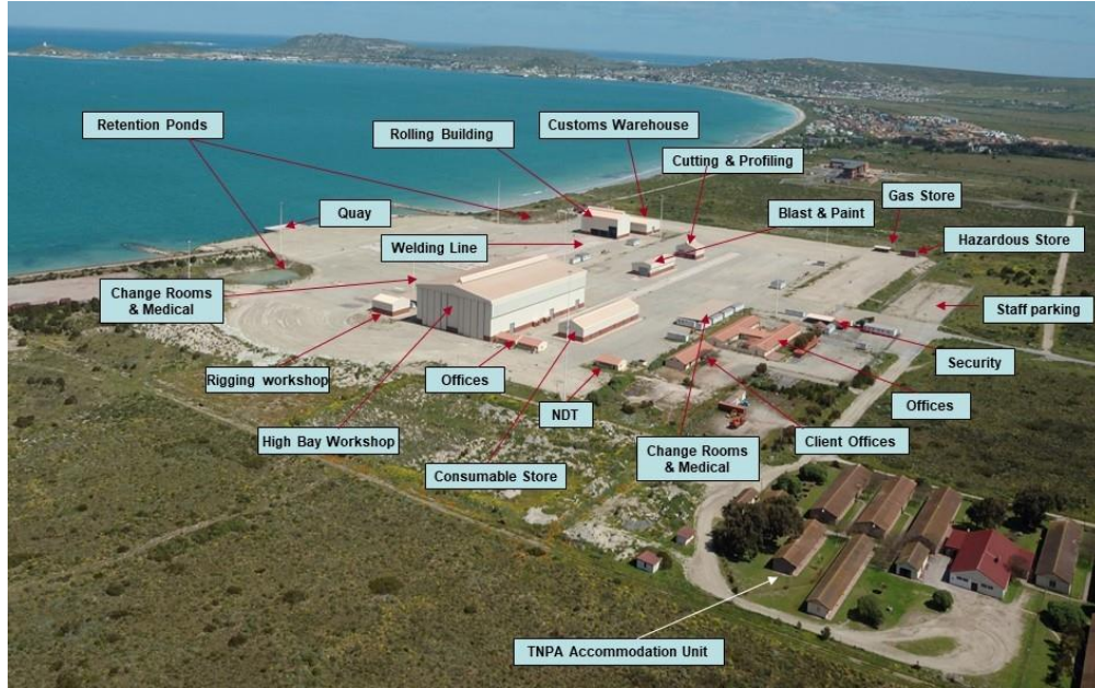
Figure 4: Moss gas Fabrication Facility Port of Saldanha development post-2007
